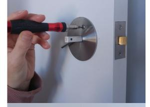
12. You may unscrew the lock snib and install it onto the preferred side (if required). Ensure that you unlock the unit first before removing it.
