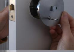
8. Now screw in the first securing bolt (M4 35mm)
