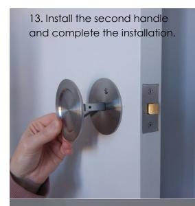
In an emergency, a locked handle can be opened from the other side.
